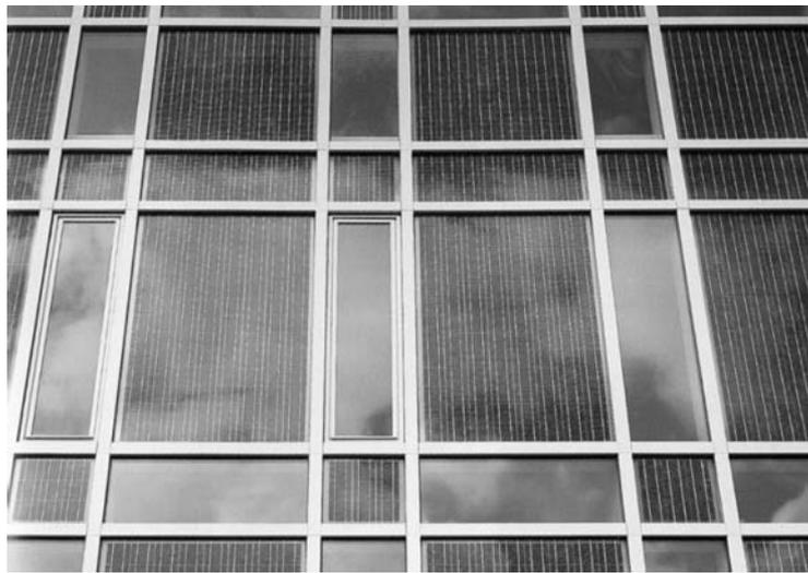
**Fig. 10.11.** PV-façade equipped with multi-crystalline PV modules and windows in a chess-board type of arrangement (seen at “Stadtwerke Aachen”).
