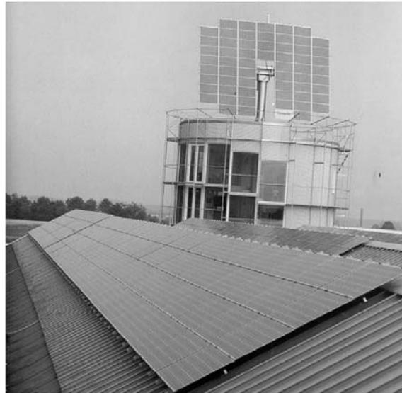
**Fig. 10.1.** Fixed mounted PV modules and 2-axis tracking of a 6.6 kW<sub>p</sub> PV generator (Hans Grohe, Offenburg).
