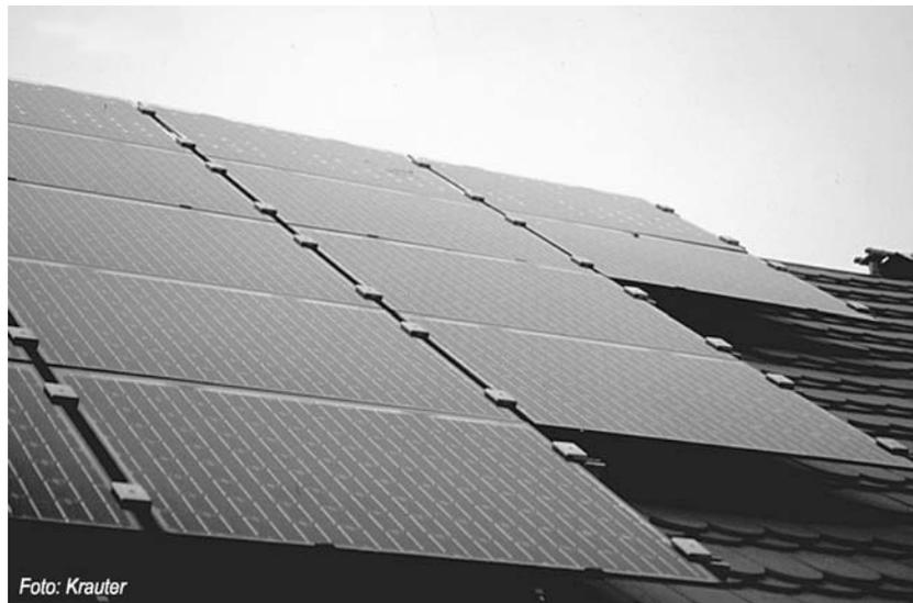
**Fig. 2.16.** Roof-mounted PV generator with frameless modules and fixture compounds.
