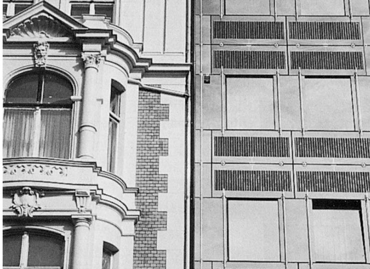
**Fig. 10.12.** PV-façade at the Ökotec-building in Berlin-Kreuzberg (right side) in conjunction with a historic façade from the “Gründerzeit” (left side).
