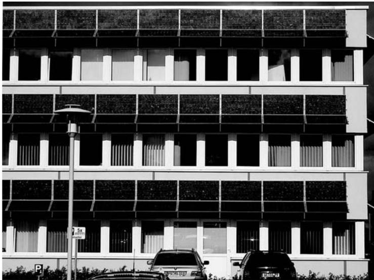
**Fig. 10.13.** PV-façade with PV modules as window shading elements to reduce air-condition load and glare (seen at Solarworld in Freiberg, Saxony).
